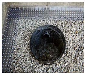
The Hydro-Channel installed overlapping onto a 4 inch clean rock subgrade which will allow the system to drain into perforated sump container.
