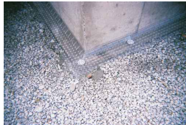
Inside corner installed
