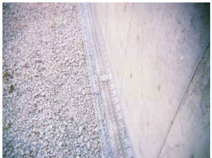
View of track overlapping footing onto the 4 inch subgrade
